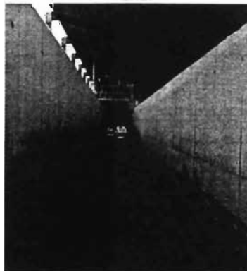
Emptied bay awaiting intake of new material for composting
