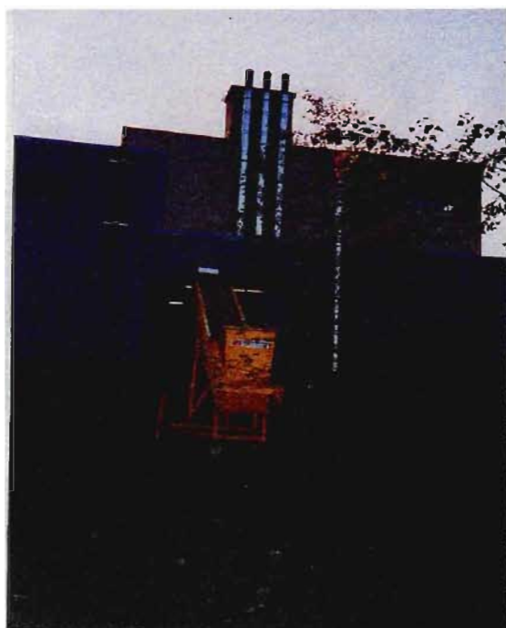
Small (100 kW) combined heat and power unit at Enniskillen College, Co. Fermanagh
